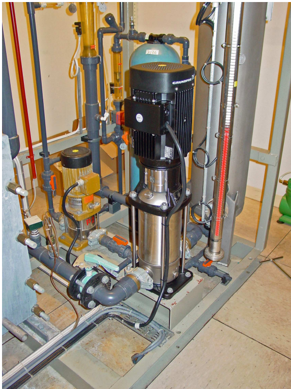
The new pump for water cooling of the cyclotron
